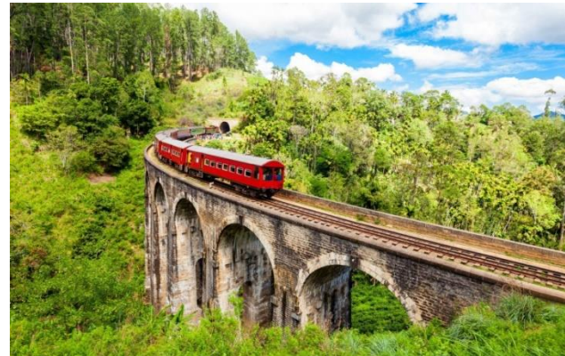
Nine Arch Bridge
